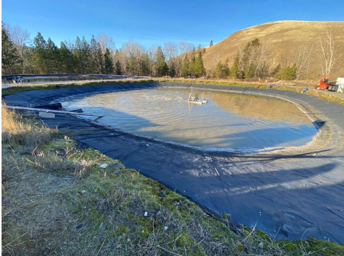
Figure 2-6. Equalization Basin
