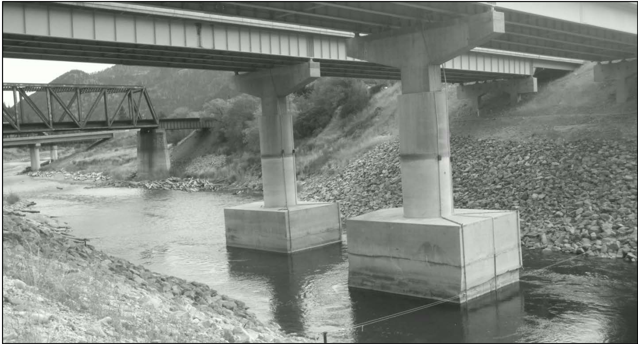
Figure 3-8. View of I-90 bridges and retrofitted center piers in Blackfoot River.
