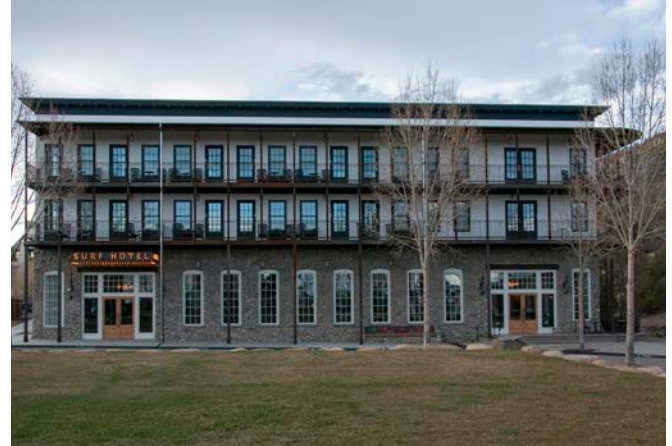
Larger and more prominent buildings can be located closer to West Broadway Street.
