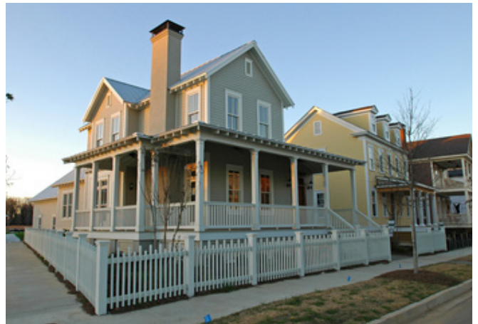
A large single family detached house with porch. A picket fence marks the Frontage Line.
