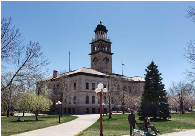
Greater design flexibility allows buildings to be sited in locations of particular geometric importance.
