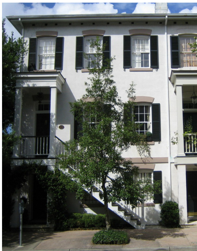
Figure 5-19: An at-grade entrance, and an exterior stair leading to the entrance of the unit above
